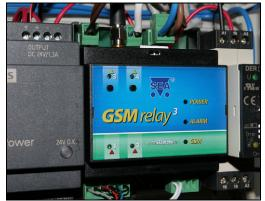
GSM relay to enable remote control via cellphone.
